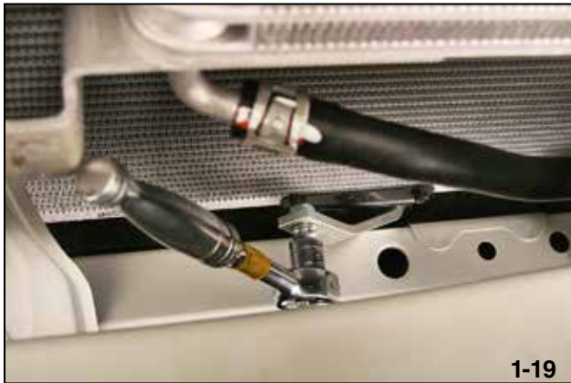
Removing Lower Bolt
