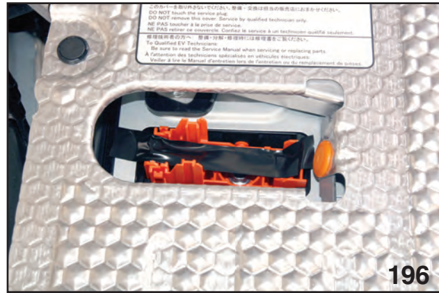
Tape Exposed Terminals
