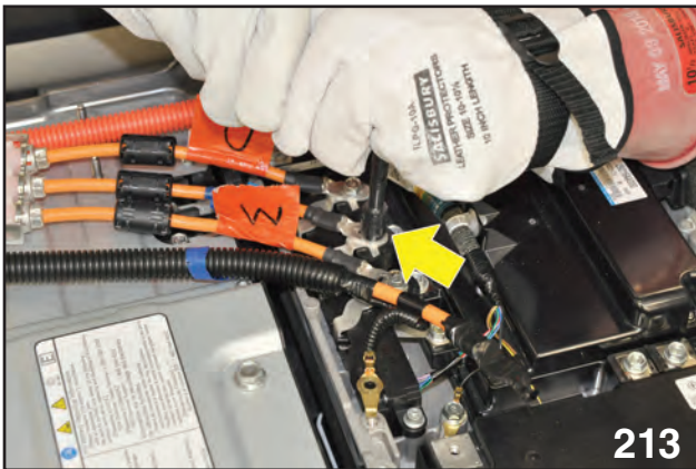
Removing Motor Wires
