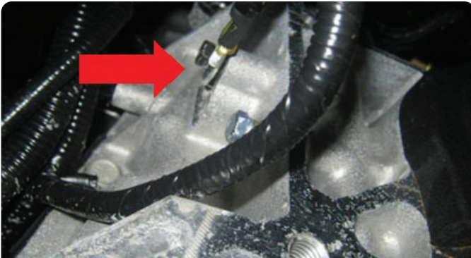
Check for a loose ground at G113.
