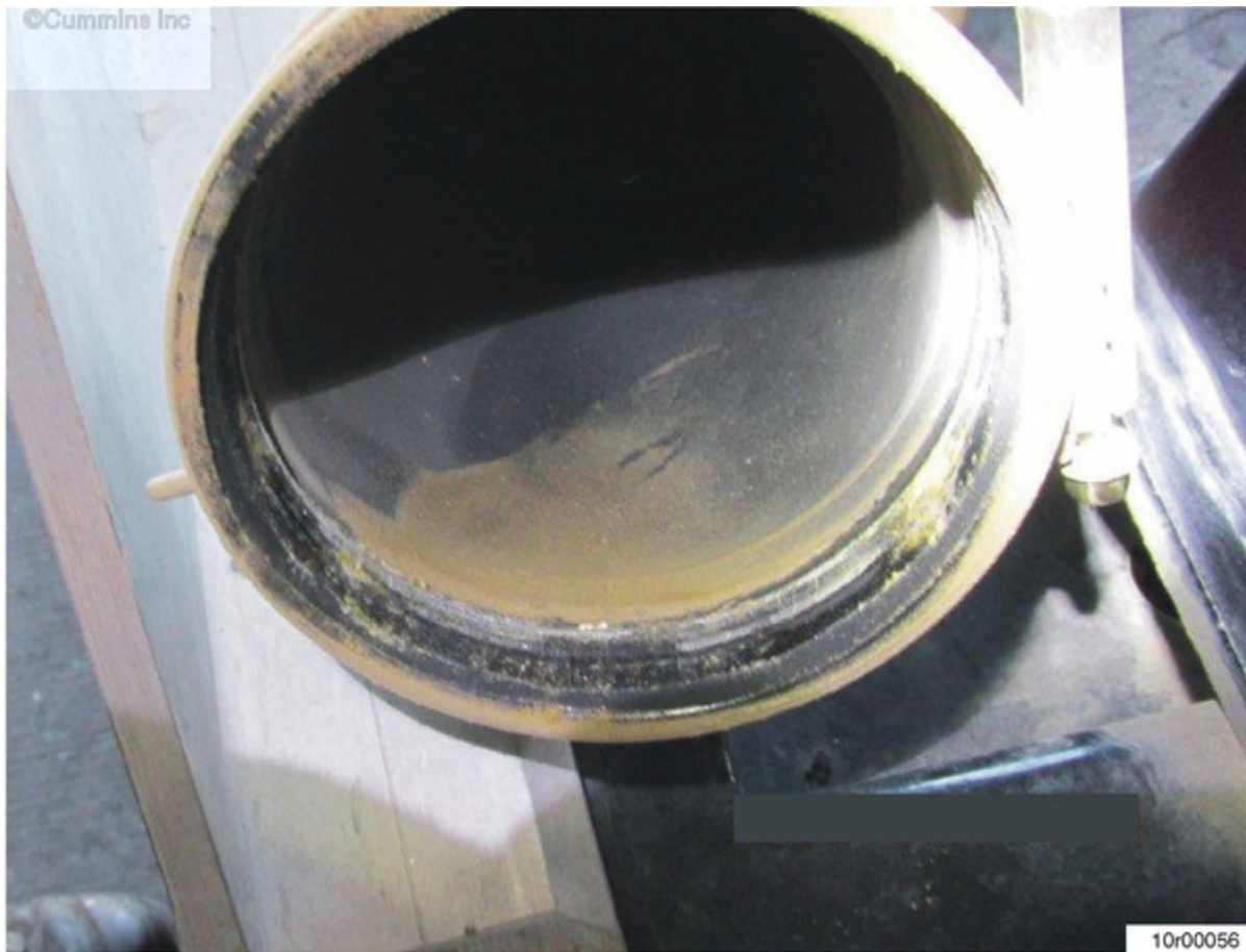
Figure 4: Dust and debris entering connection point at turbocharger compressor inlet.
