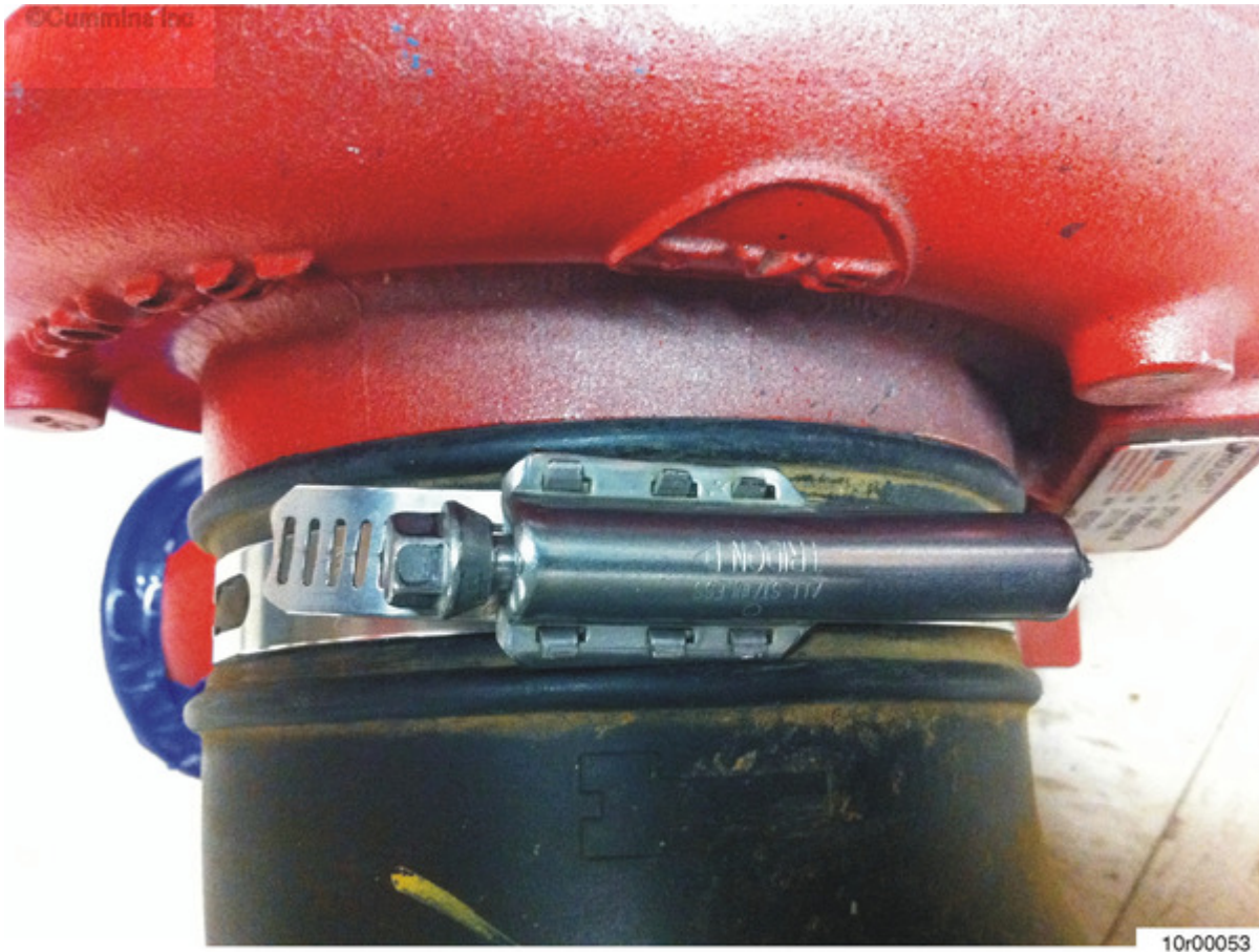
Figure 1: Gap indicating a clamp not at proper torque.
