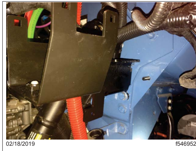
Fig. 4, New PTPDM Bracket Installation
