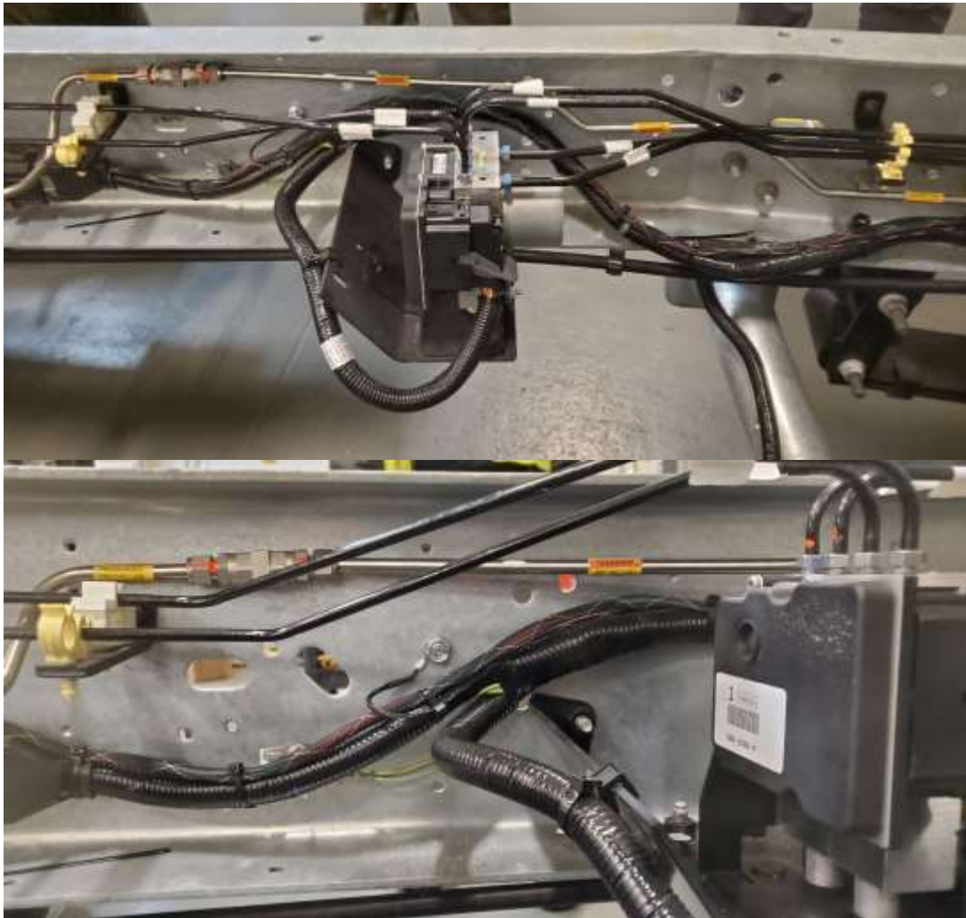
Figure 9: New ground harness secured to chassis harness.
