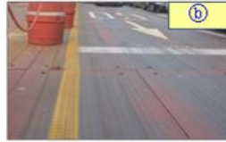
● Steel floor (subway construction site)
