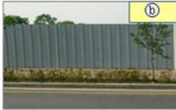
● Iron wall at the construction site
