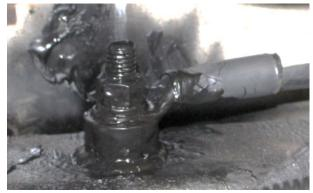
FIGURE 80: GROUND STUD WITH RUBBER COATING
