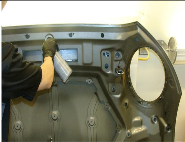
14. Using the remaining ½ of the bottle of cavity wax **remover**, apply again from the top down. Repeat steps 11 through 13.
