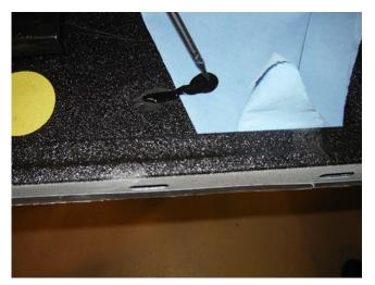
6. Noting the viscosity of the repair material, moving from the towel to the repair area, use a slow bead to fill the entire repair area from the outer edges, spiraling into the center moving back to the towel leaving no tail of the material on the repair area.
