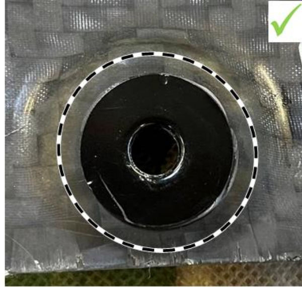
Figure 4 (areas are not corroded = OK)
