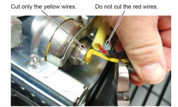
• Strip away about 1 inch of the yellow wire insulation, then twist the wires together.
