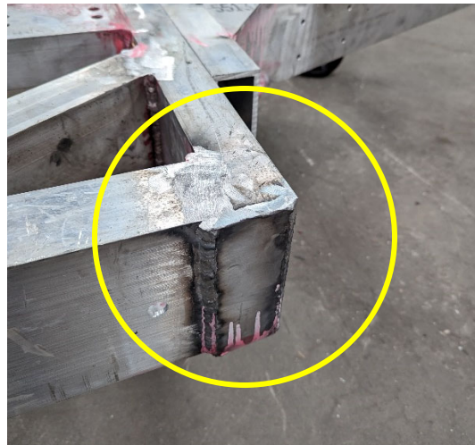
Figure 2) Welds on the front curbside corner of the frame
