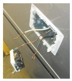
Loosen the silver and brass screws to remove the black and white wires from the receptacle.
