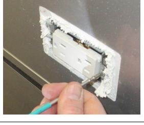
Remove the two receptacle mounting screws.
