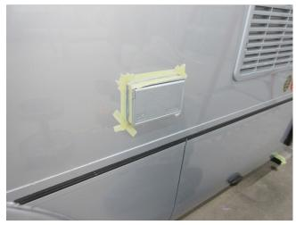
Touch-up paint around the receptacle if necessary.
