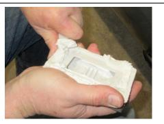
Remove Butyl from cover and sidewall with the plastic windshield tool.
