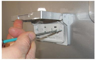
Remove the two receptacle cover screws. Put screws aside for later
