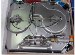
7. Visually inspect the gas tubes connecting the gas valve to the burner orifice holder for any cracks, splits, etc. Ensure no gas lines are loose by <u>gently</u> pulling the tubing along its axis away from each brass nut. <u>Use only two fingers.</u> If any gas lines are loose, stop the recall kit process and request a replacement unit by contacting Suburban Tech Support at 574-247-9235, option 5.
