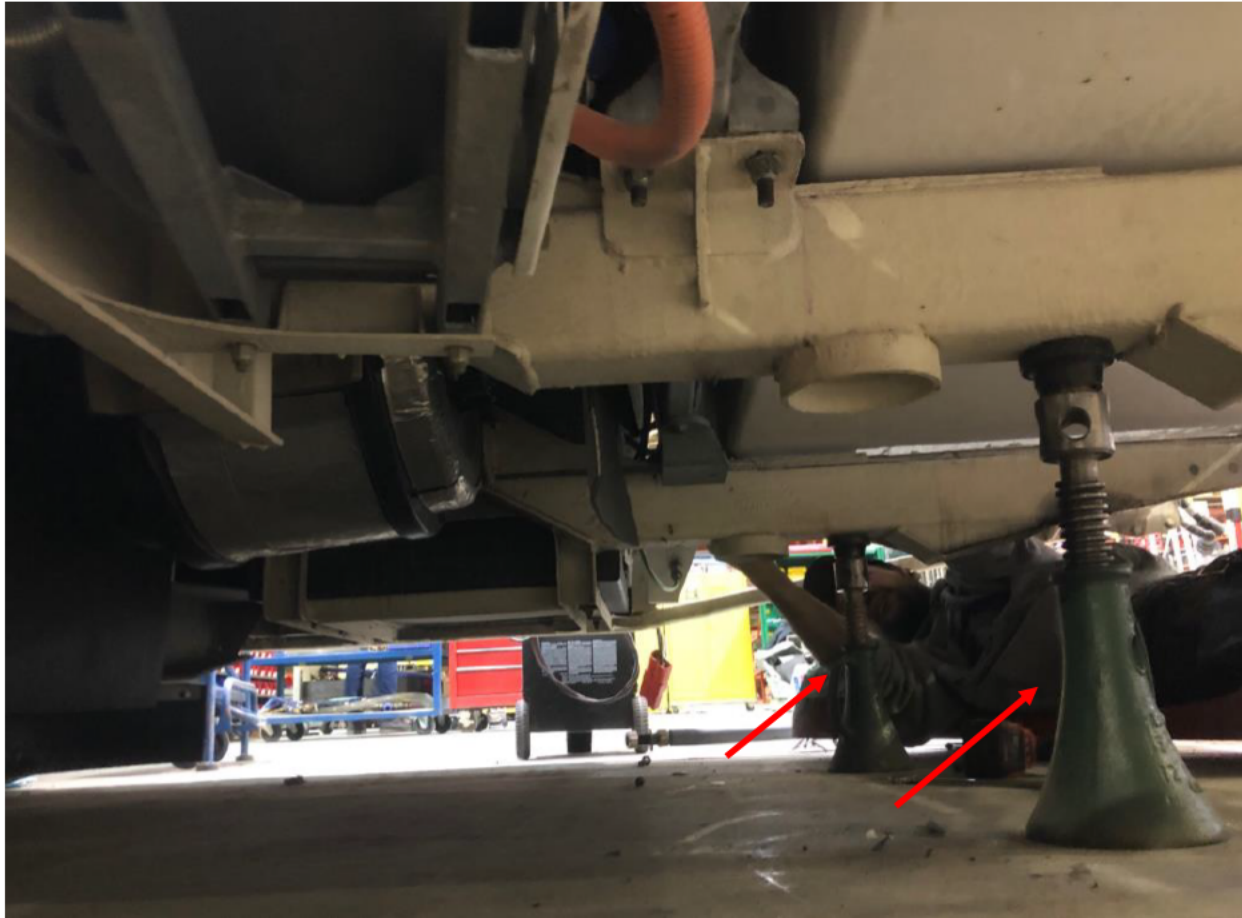
Figure 3: Support Rear Frame Members with Jack Stands
