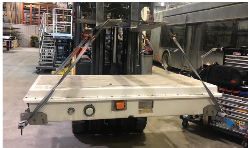
Figure 16: Lifting Upper ESS Enclosure
