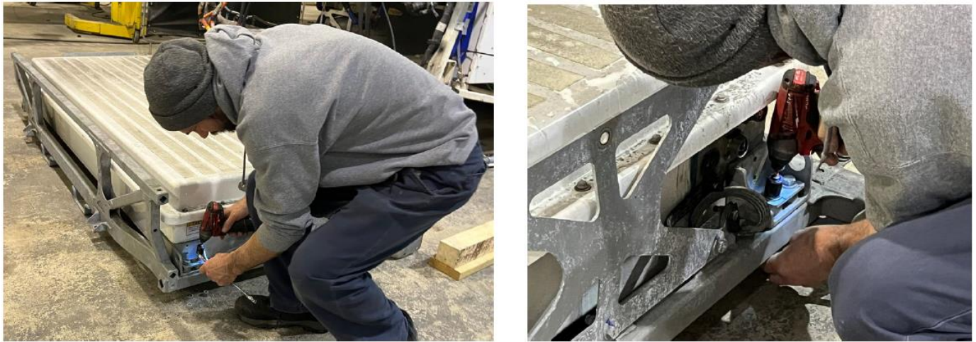
Figure 17: Removing Hardware from ESS Enclosure Feet
