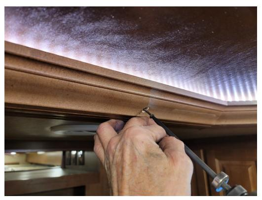
5) Glue wood buttons into the drilled 3/8" holes.
