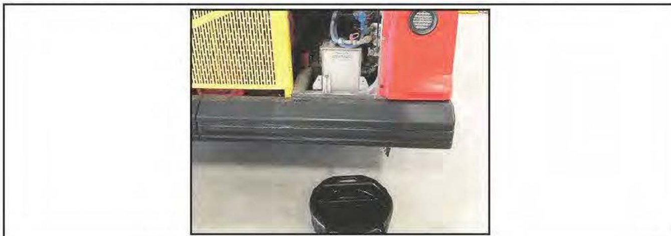
Figure 1 - Place Container to Collect Hydraulic Oil
