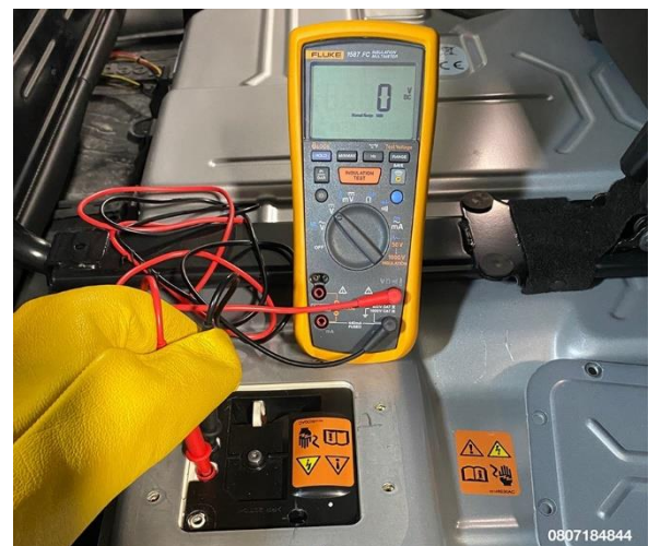
Figure 6 – Measuring at High Voltage Test Points
