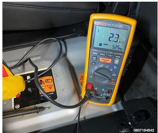
Figure 11 – Measure and Record Isolation Resistance Between HV Positive Test Point and Chassis Ground
