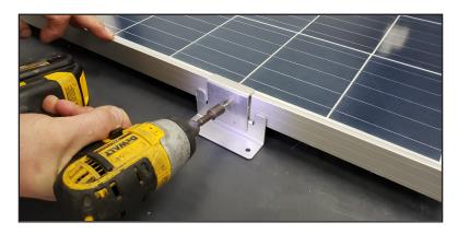
5. Drill out the other two holes on the add-on bracket and through the pre-existing mounting bracket.
