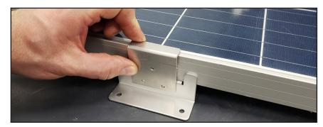
3. Drill a hole (using the 3/16 size drill bit from the kit) through the L-bracket pilot hole and the solar panel. Drill into the panel as straight as possible. Drilling at an inclined angle could result in hitting the M6 fastener of the pre-existing bracket behind the panel frame.
