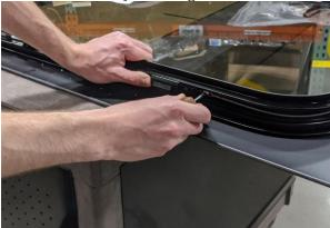
Figure 21a: Installation of ER bar screw.
