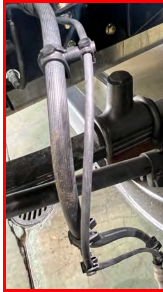
Figure 3 - Tire abrasion/Damage on Hose
