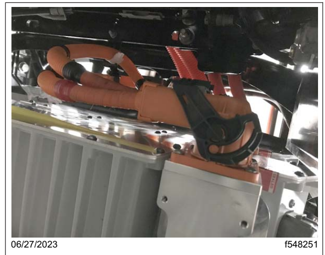
Fig. 3, High-Voltage Cable Connection Location
