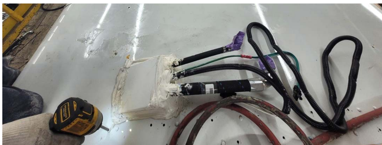
Fig. 14, Installing the Screws along the Joint
