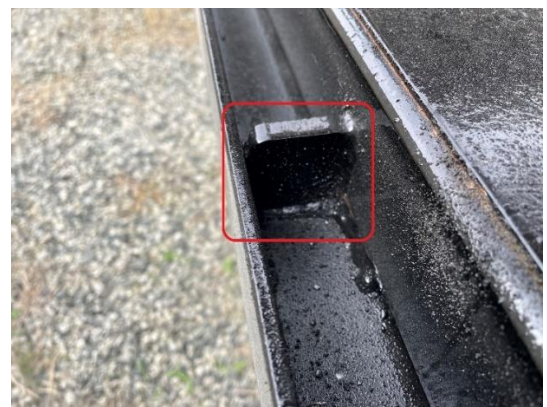
Properly Installed Angle Ramp Track with Caps, Gussets and Welds
