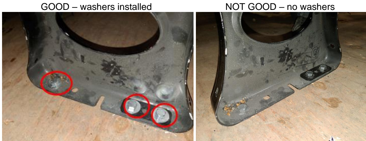
Figure 1: leg inspection for washers
