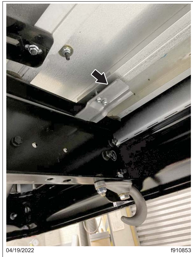
Fig. 15, Behind Rear Bumper View
