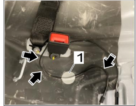
Routing the wire harness for the seat-belt buckle
