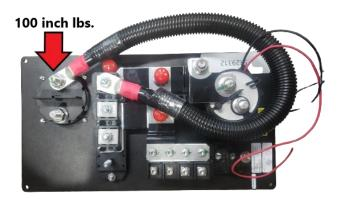
10. Loop the harness around behind the board, and connect the other end of the cable to the stud for the 400A Zcase fuse. This will require using the torque wrench set on 100 in lbs.
