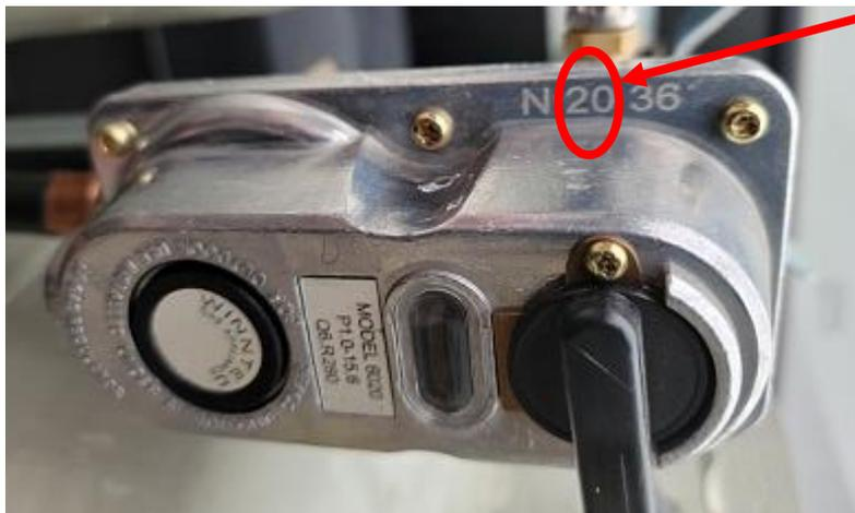
Because the first set of numbers in this date code is 20, the regulator must be removed and replaced in accordance with this recall.
