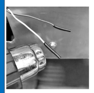
Install heat shrink cap (K) on each of the wires and use heat gun to seal.
