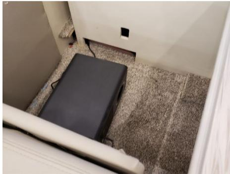
4. Pull the Romex wire from the hole. This wire should be labeled "OUTLET."
