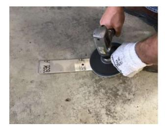
Prep the mating surface of the Aluminum plate using 40 grit nonstearate paper, and follow up with a thorough Accetone or Alcohol wipe.
