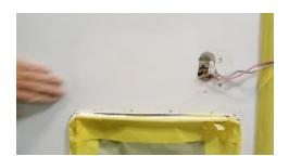
F. CLEAN OFF THE AREA WITH AN AIR NOZZLE AND PRIME THE AREA;
