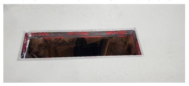
15. Prep vent using 1/2" by 1/16" butyl tape making sure to cover all screw holes. Be sure to remove wax paper before installing.
