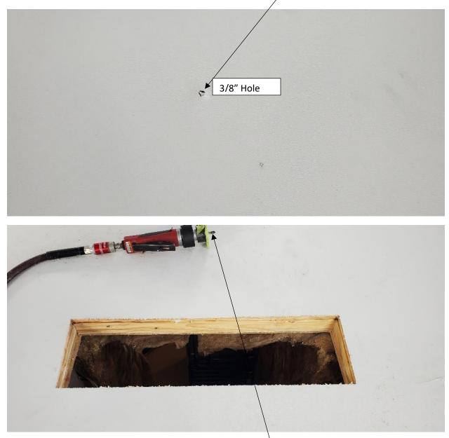
13. Make sure your router bit extends past the base at least  $1/2^{\circ}$  to ensure it gets all the way through the decking and doesn't slip out. Carefully trace opening with router being cautious not to slip or over rout.
