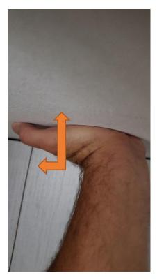
11. Once interior panel has been routed out, drill a 3/8" hole through roof decking from inside out.
