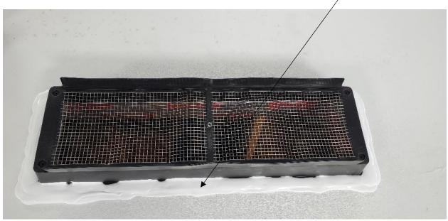
17. Install cover using four 1-1/2" #10 wood screws. Once you have secured cover fill holes with self-level sealant.
