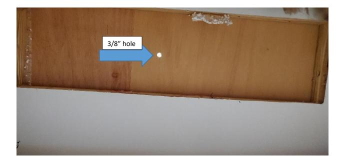
12. Once you have a 3/8'' hole from inside out, go outside the unit to the roof. Locate 3/8'' hole and rout using a pin router or similar with a new/sharp router bit.
