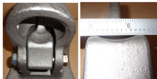
CORRECT LOCKING MECHANISM INTERNAL LOCK HAS A RADUIS
