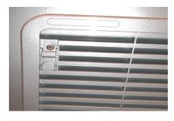
Push both tabs down and reinstall the top clip screw of the vent (start screw by hand into the metal clip on the vent frame. (Be careful not to strip the screw.)
