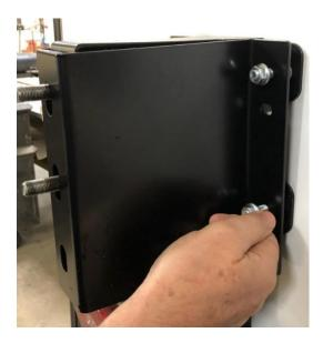
4.) Once all of the 3/8"-16 nuts are started, use 9/16" deep socket and tighten nuts to 30 ft.-lbs. against each Z-bracket.
