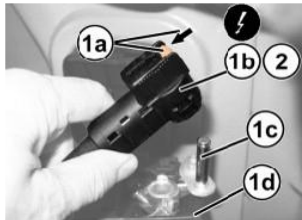
Figure 37 – Battery Negative Cable
