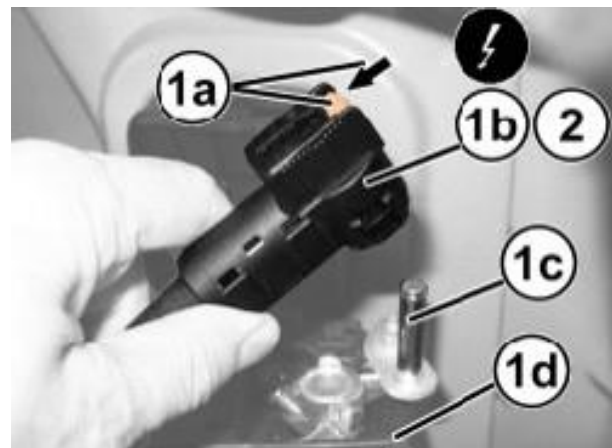
Figure 37 – Battery Negative Cable
