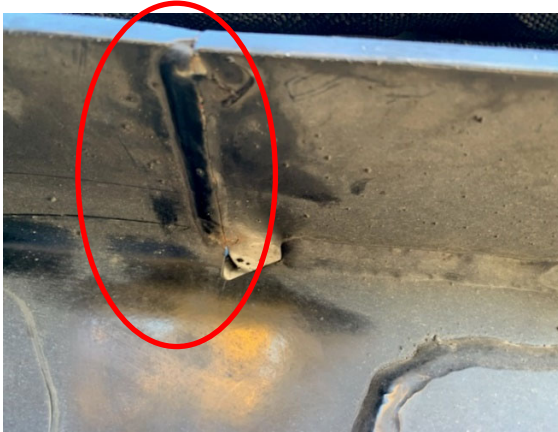
Photo 5 Crack example: frame horizontal top
