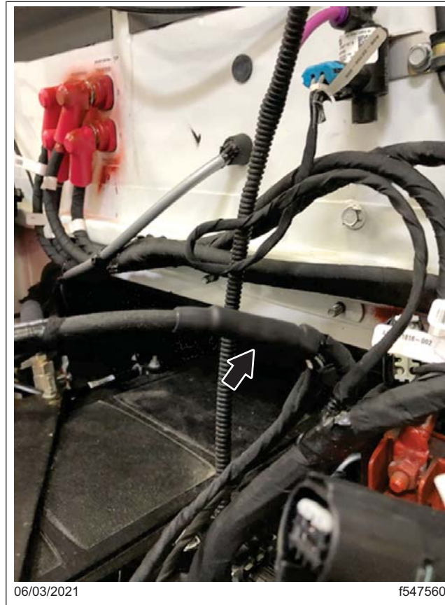
Fig. 17, Heat Shrink Applied to the Splice
