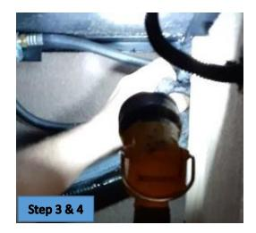
5. Remove the furnace cover. You will need to remove the exhaust (#1) prior to removing the cover (#2). Set all parts and screws aside for reuse later.
