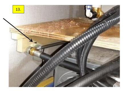
Using a 3/4" open-end wrench, install the furnace connection to the manifold extension connection (#14).
