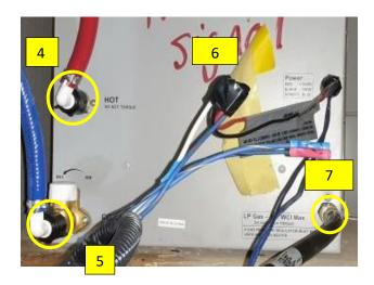
28. Add foam sealant (in the storage compartment) around the newly installed LP hose replacing any foam that was taken out when removing the original hose (#18).
