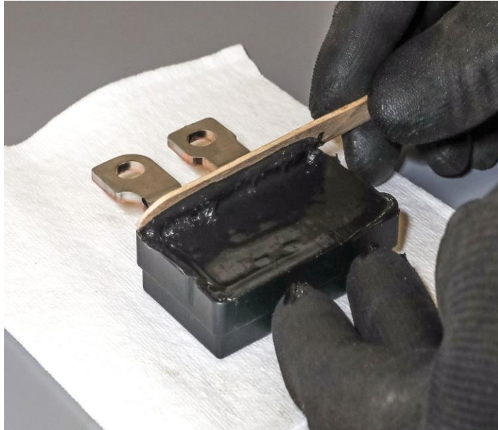
Figure 5 – Skimming Excessive RTV
