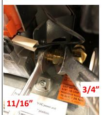
Remove elbow from water heater with a 11/16" wrench holding at the heater and a 3/4" wrench on the fitting.
