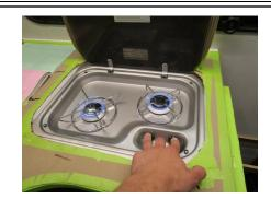
Ignite the stove top and allow it to self extinguish to burn off existing propane in the lines.
