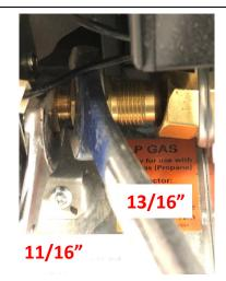
Remove the connector by holding the fitting at water heater with a 11/16" wrench and a 13/16" wrench on the coupling.
