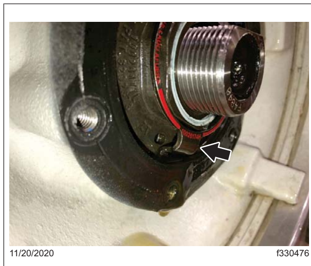
Fig. 4, Lower Snap Ring Tab is not Fully Installed in the Spindle Nut Locking Hole
