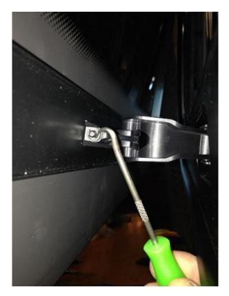
4. Remove the pin that secures the latch to the glass.
