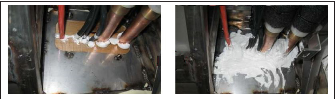
Figure 16 - Cover Blocks with White Sealant SikaFlex 221
