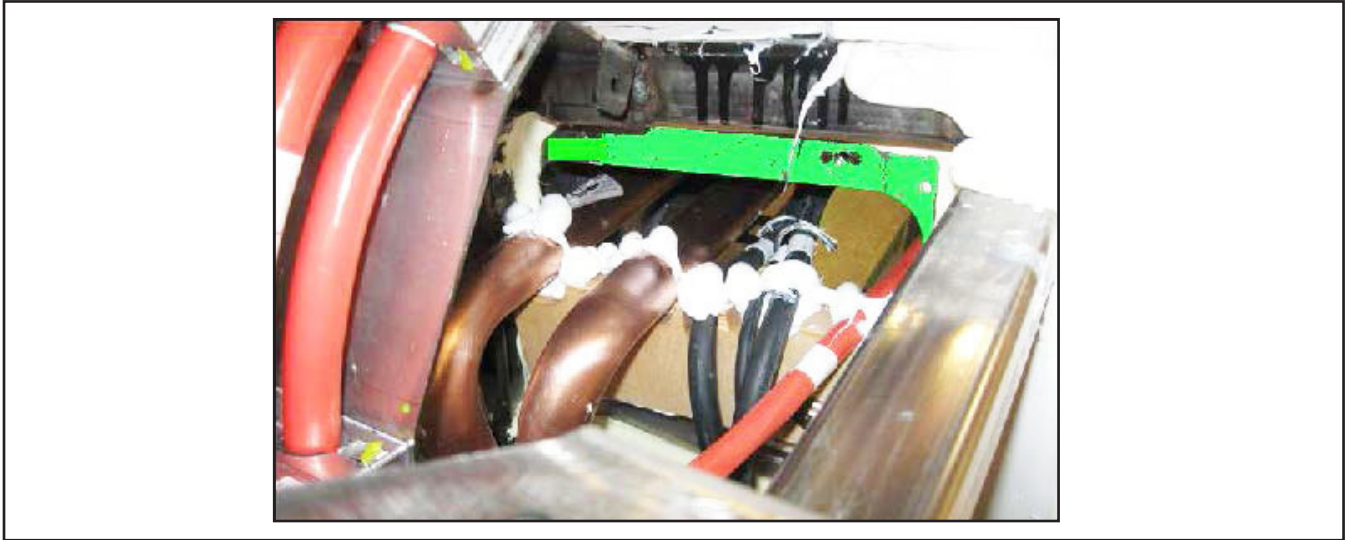
Figure 13 - Apply White Sealant SikaFlex 221
