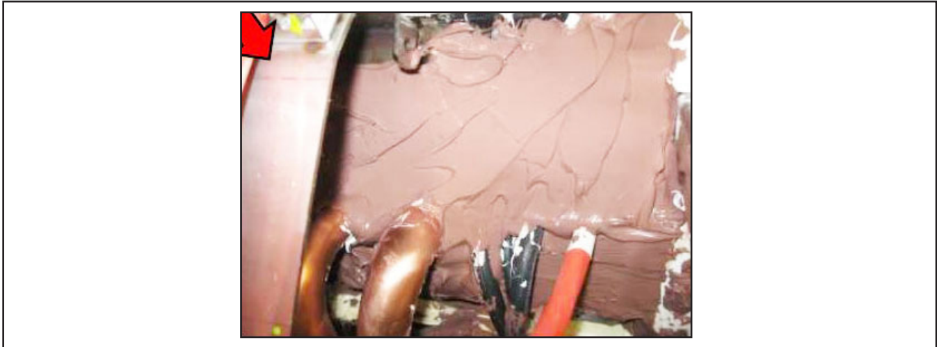
Figure 17 - Cover Blocks with Fire Stop Sealant
