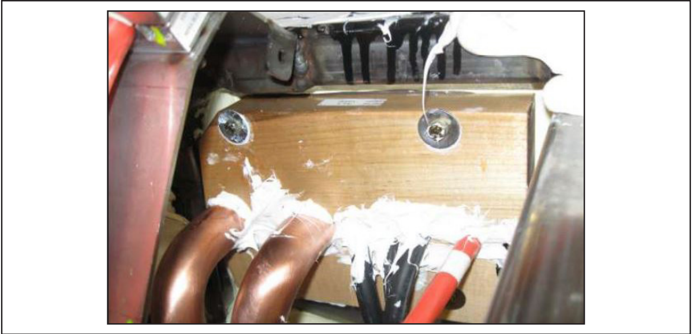
Figure 15 - Verify the Sealant Application
